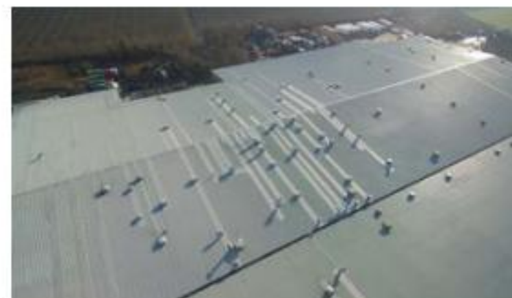
Delcote/Seamsil Project 32,500m 2 roof Spade Lane, Sittingbourne
